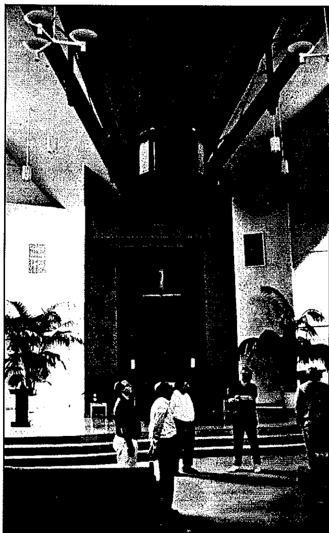
FIGURE 4-8. Type 1B central cluster system comprising four Renkus-Heinz TC-3 RPA reference point array loudspeakers at the Irvine Presbyterian Church in Irvine, CA. System design by Ron Sauro of Northwest Audio and Acoustics. Photo courtesy of Renkus-Heinz.
