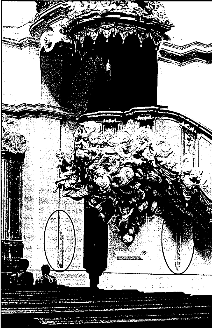
FIGURE 4-24. Type 3A standard column loudspeakers at the Katholische Hofkirche in Dresden Germany. System designer not known. Note low position of the column loudspeakers to the seating area necessary to maintain high D/R ratio. Photograph courtesy of Ihlow.
