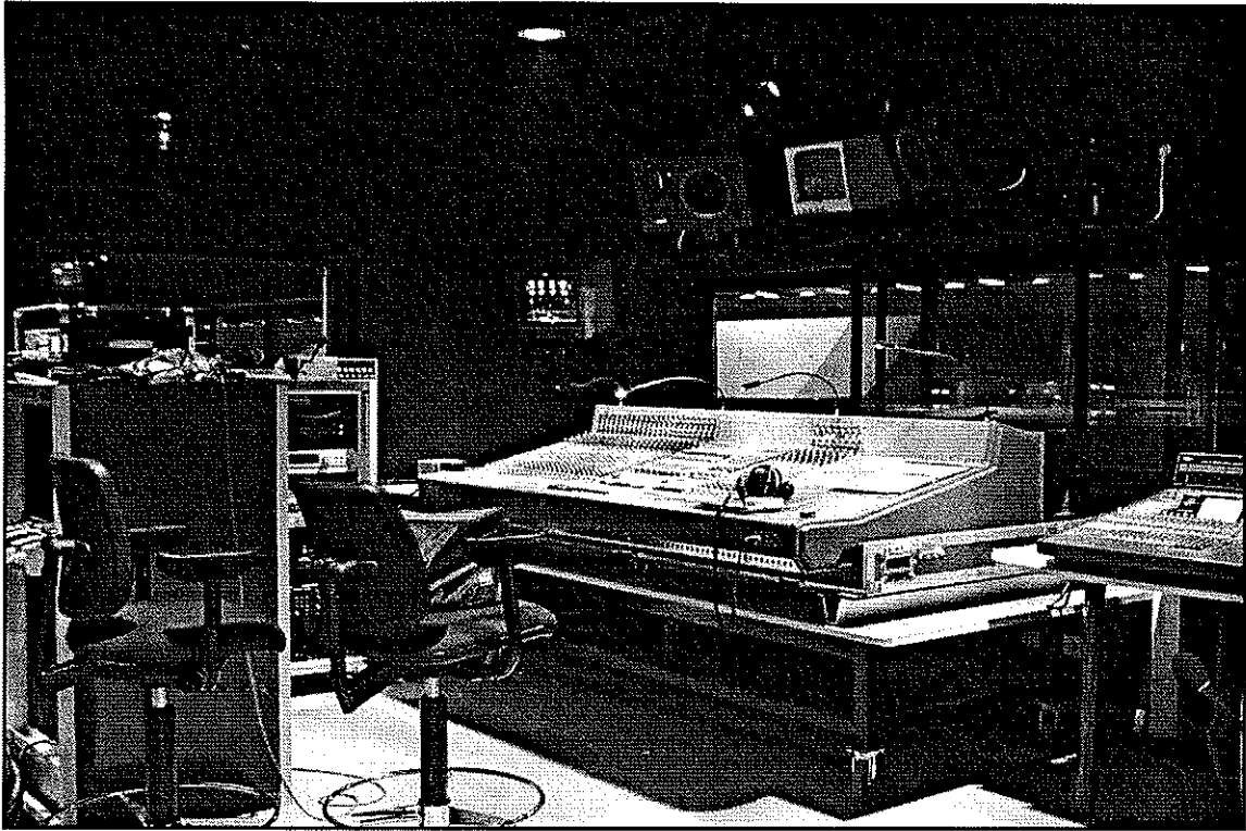
FIGURE 7-9. Large audio control room in the Auditorium de Dijon in Lyon, France. Note MIDAS XL4 mixing console on rolling table (left), Yamaha 02R digital mixer (right), Genelec monitor loudspeakers, and Panasonic video monitor all above operable control room window. Control room walls and ceiling are painted black. System design by Tom Young of ARTEC Consultants, Inc. Photo courtesy of ARTEC Consultants, Inc.
