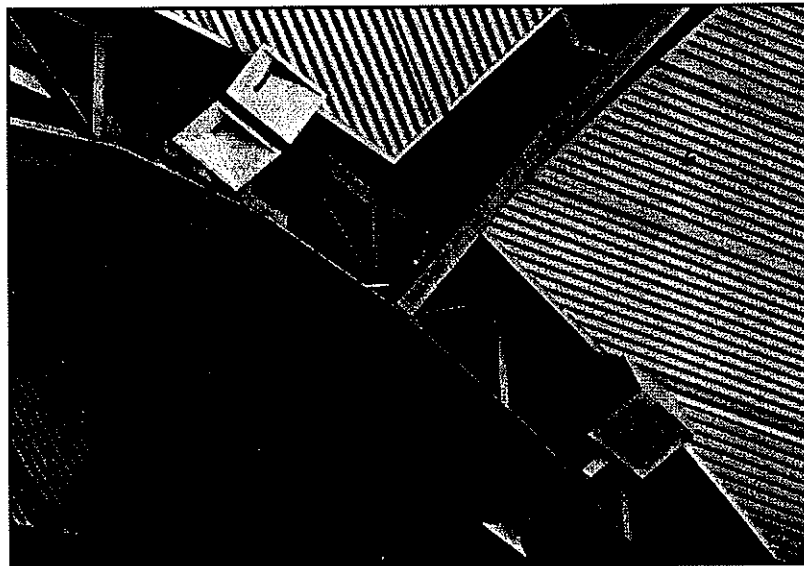
FIGURE 4-16. Widening of loudspeaker coverage angle by cross-firing in the vertical plane small format constant directivity horns (Electro-Voice 640 with DH1A compression driver) and 12 in low-frequency driver (in custom enclosure) at Reagan National Airport in Washington, DC. Note the small low-frequency enclosure at the opposite side of the horns. Low-frequency cabinets are arranged with the driver facing the opposite horns. Omni-directional nature of low-frequency sound permits this installation concept. System design by Bob Ledo of Coffeen Fricke Associates.
